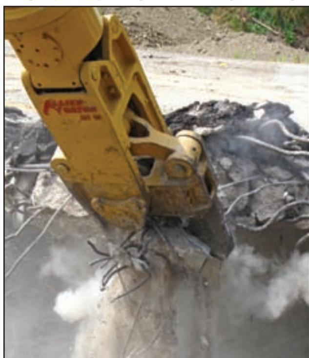
B.O.G. demolishes thick concrete on the Cadiz bridge with the MTR 50 C.
