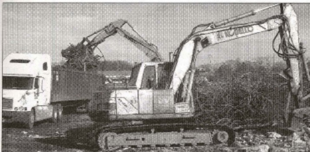
E. Luke Greene Co.'s 130 Kobelco equipped with a Wag Way Concrete Crusher downsizes concrete and separates rebar, while a second excavator loads scrap steel.
