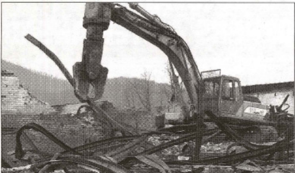
The Allied-Gator MTR70 is frequently used on demolition jobs that require the company to remove steel and concrete buildings. The MT series Multi-Tool is used to tear through the material within a structure, removing large pieces one at a time and later, reducing the steel and concrete to smaller-sized pieces for ease of transportation.
