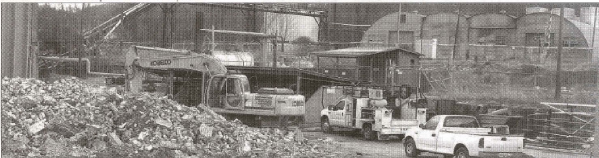
Just part of the equipment used in this demolition project.
