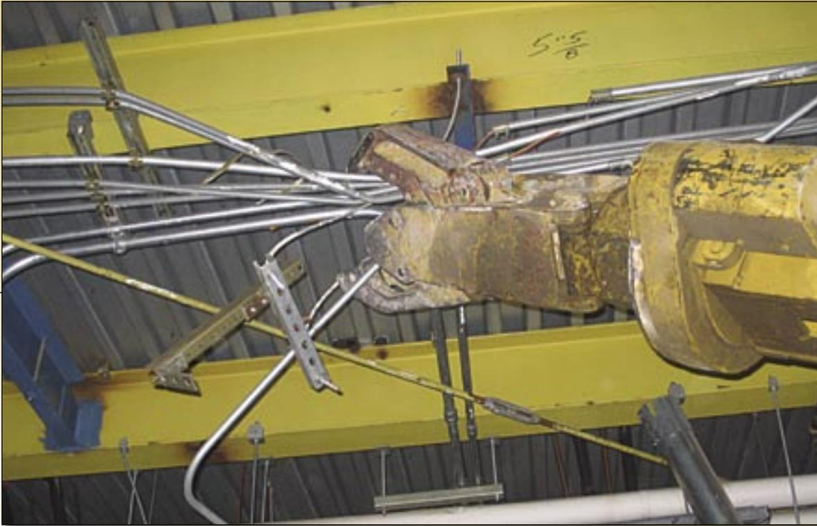
design allowed them to provide a small tool that could be mounted on a mini-excavator. Additionally, they could offer a third member configuration that would afford Watral the ability to reach, rotate, remove and process targeted materials easily. This configuration would also allow him to virtually eliminate the use of man-lifts and substantially increase productivity.
